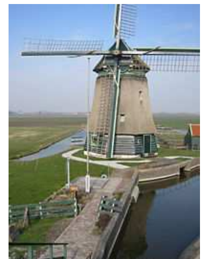
POLDERS IN THE NETHERLANDS (windmills and canals are part of the polders that remove water from land and make it suitable for farming)
